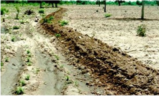
Recently installed contour bund on a farmer field in Mali
