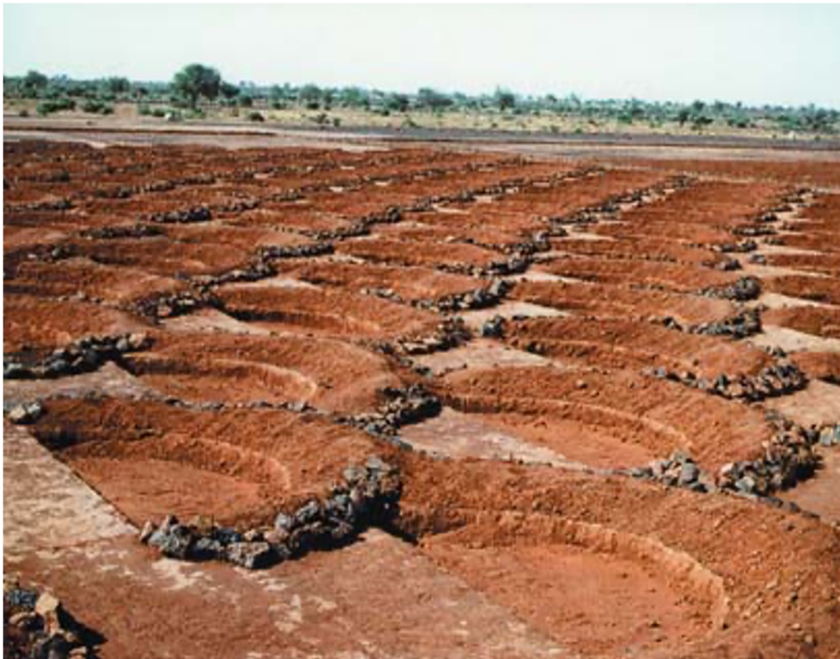
Semi-circular bunds reinforced with stones
