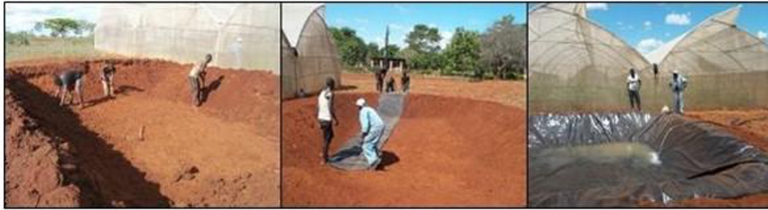
Establishing a small fishpond (left to right): 1) excavating and smoothing the pond, 2) spreading the PCV liner and burying the edges, and 3) filling the pond
