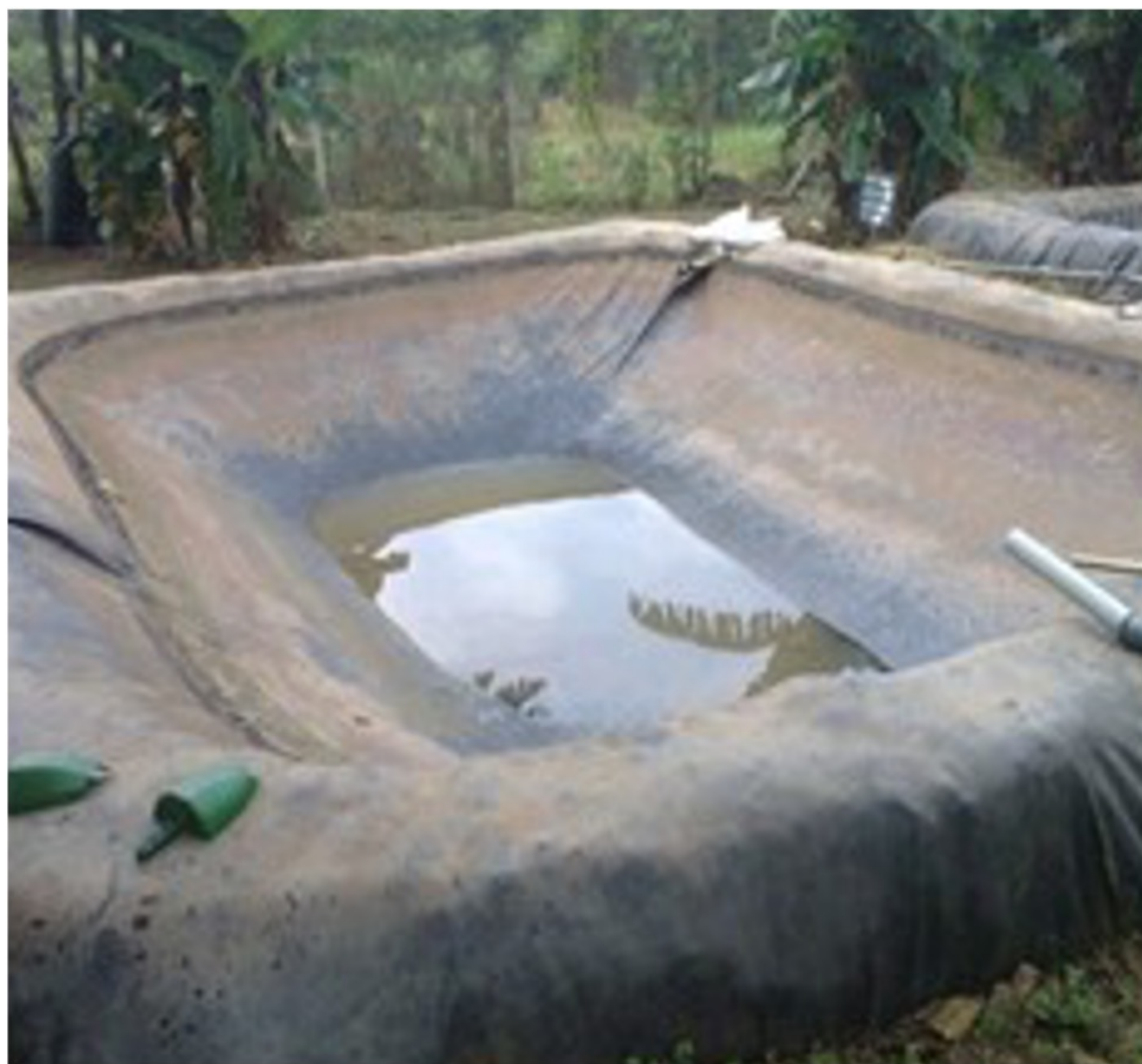
Excavated pond with liner
