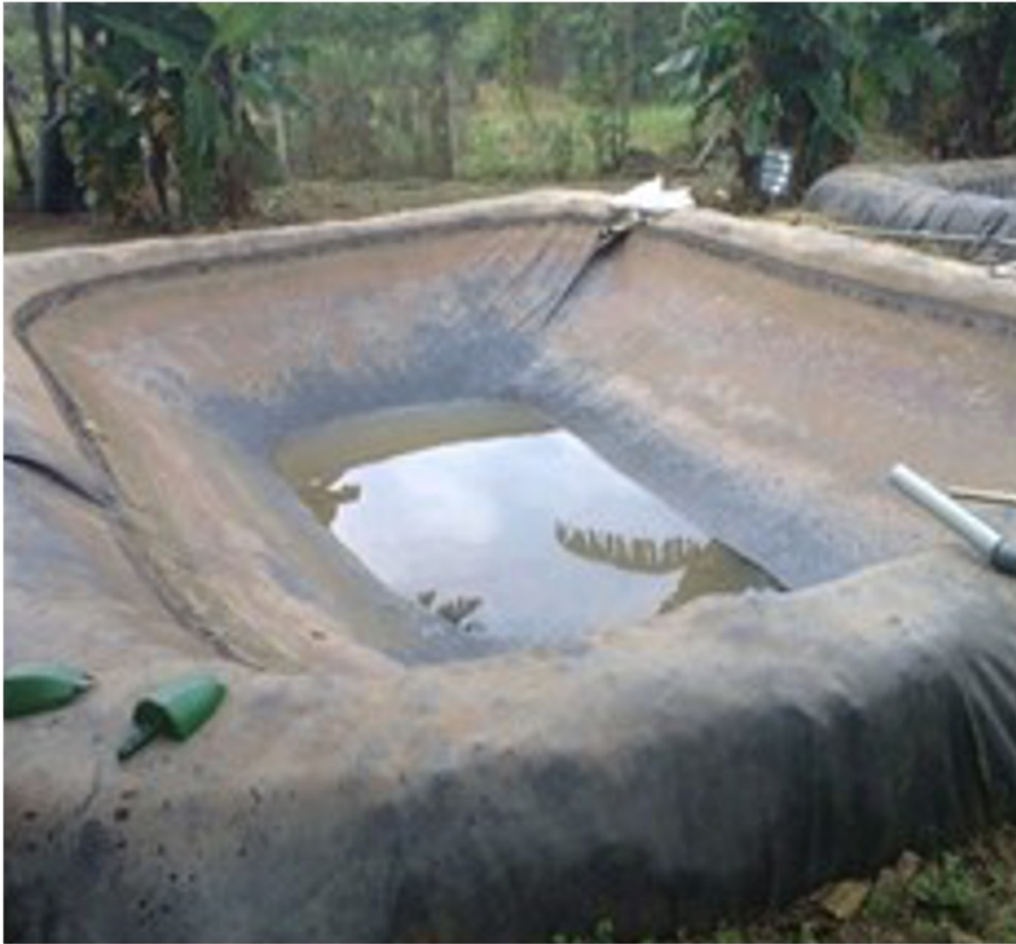
Excavated pond with liner
