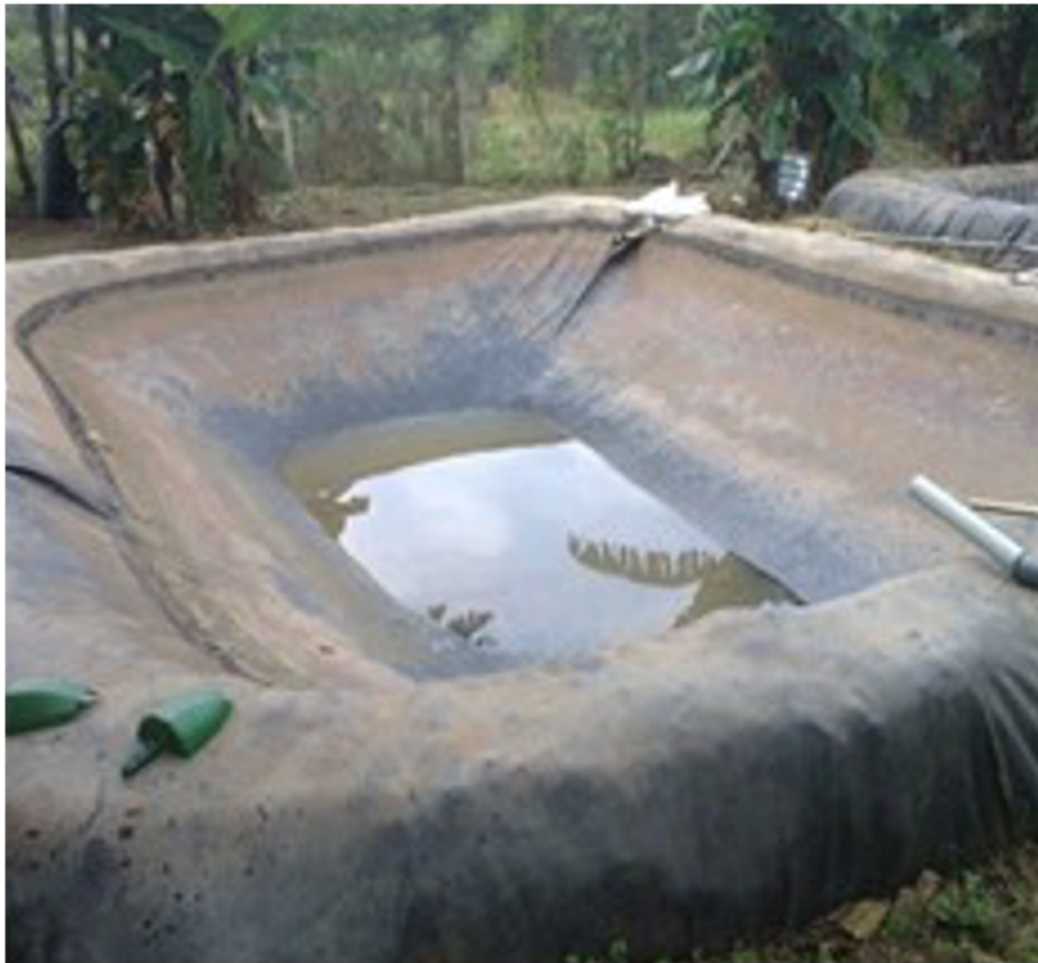
Excavated pond with liner
