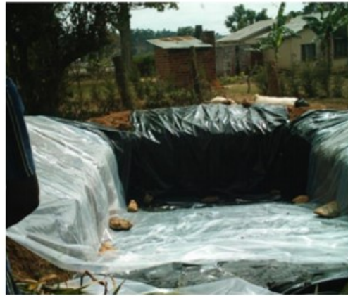
a) Digging a trench and lining it with plastic sheets
