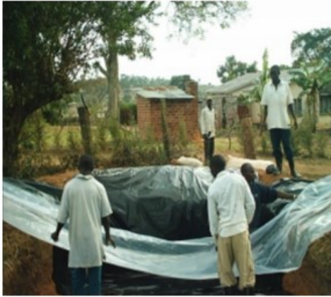
a) Digging a trench and lining it with plastic sheets
