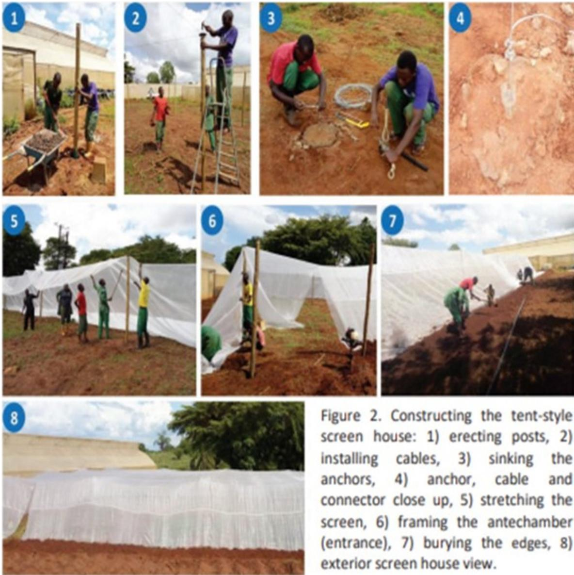
Figure 2. Constructing the tent-style screen house: 1) erecting posts, 2) installing cables, 3) sinking the anchors, 4) anchor, cable and connector close up, 5) stretching the screen, 6) framing the antechamber (entrance), 7) burying the edges, 8) exterior screen house view.
