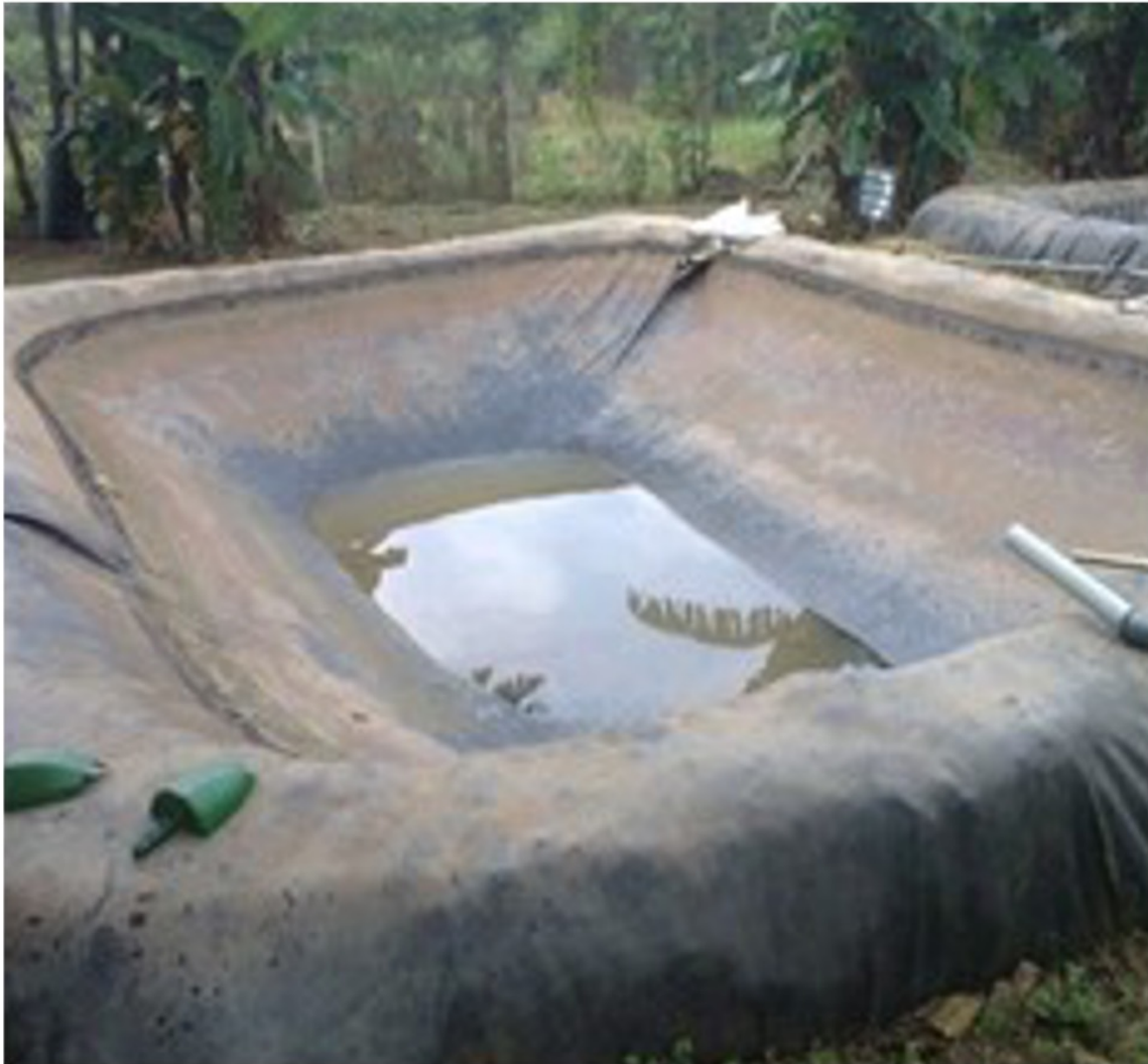
Excavated pond with liner
